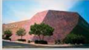
1983 Bullock's Department Store Northridge, CA, USA Building collapsed in 1993 Northridge Earthquake, tiles remained bonded.
