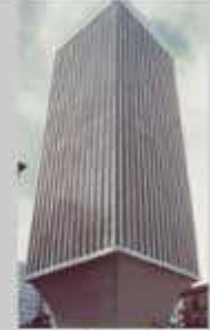
1977 Rainier Tower Seattle, WA, USA Tile base of structure subject to extreme movement
